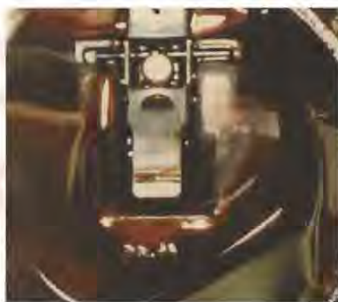
Long chain hydrocarbon buildup in a vaporizer chamber, hinders proper fuel and air blending. The normal result of running untreated LPG.
